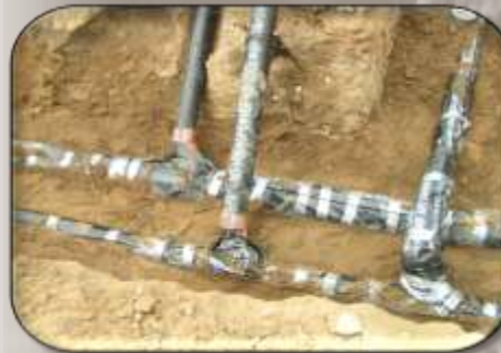
corrosion protection of buried water lines - Hospital in San Francisco
