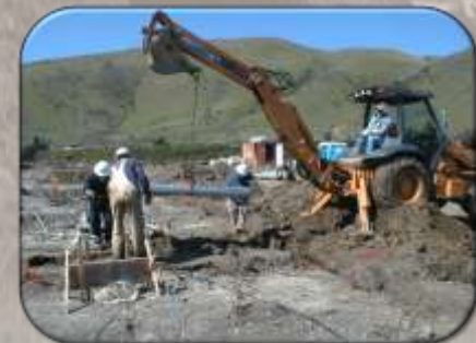
impressed current cathodic protection system installation
