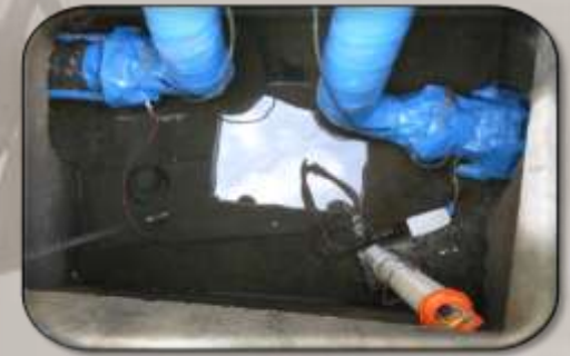
corrosion protection of buried firewater line
